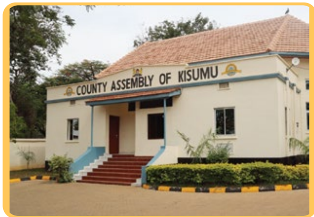
Renovated Assembly Chambers
