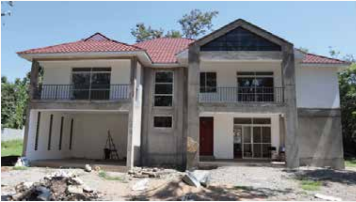
The Speaker's Official Residence under construction
