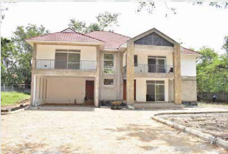
Speaker's official Residence under construction.
