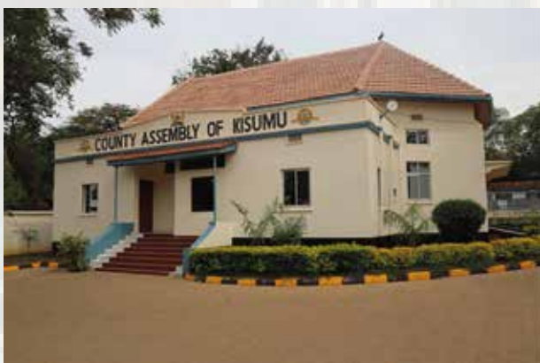
Renovated Assembly Chambers
