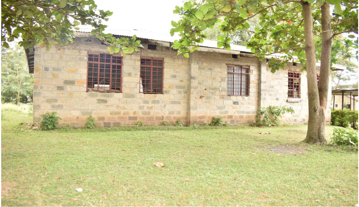
One of the condemned buildings.
