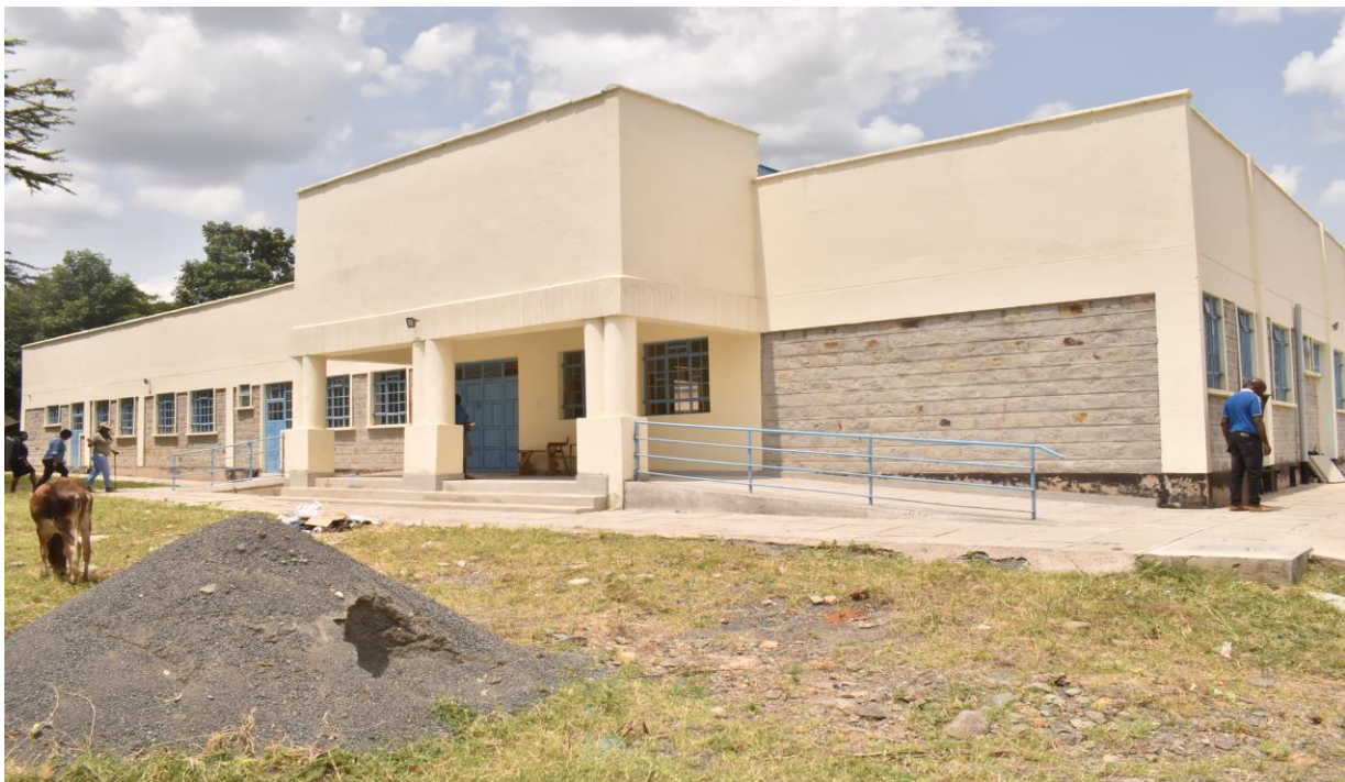
The exterior of the maternity complex under construction
